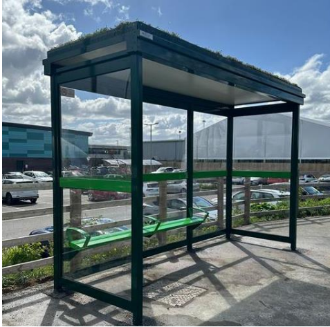
Figure 9 – Image of one of the new sedum roof shelters
